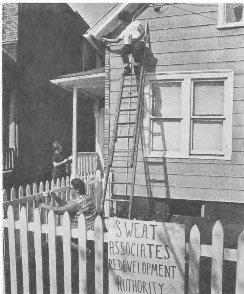
SWEAT workers apply a fresh coat of paint to the house of an elderly widow. A bill for the repairs will be sent to city housing officials.
